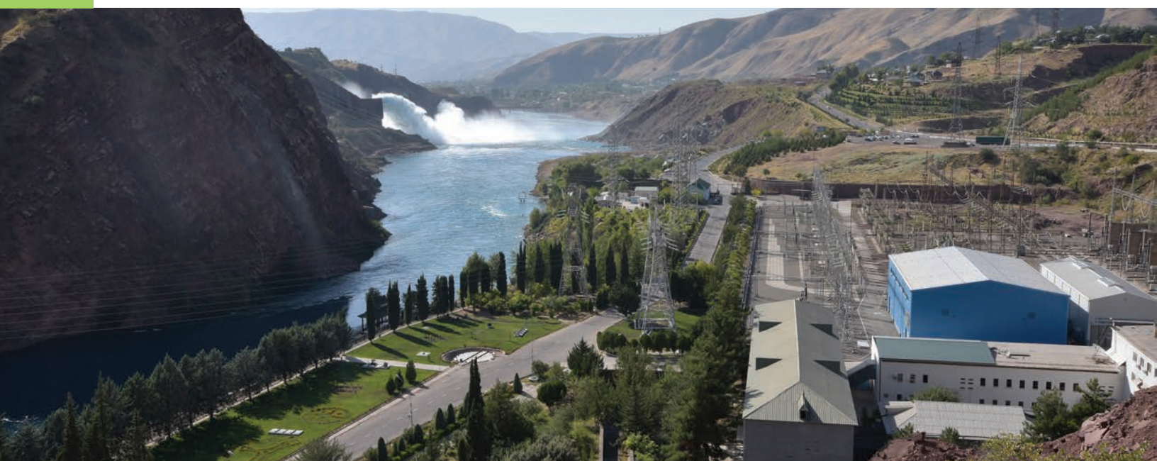
Nurek hydropower plant in Tajikistan. Photo: ADB.
