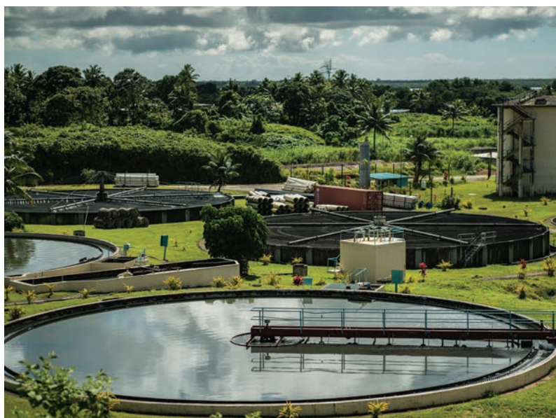
Wastewater treatment facility in Suva, Fiji. The Urban Water Supply and Wastewater Management Investment Program ensures sustainable urban growth and improved public health. It aims to provide access to sustainable water supply and sewerage services in greater Suva area. Photo: ADB.
